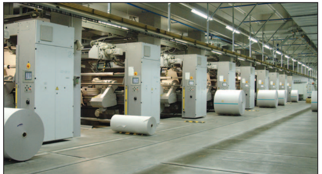
● Above from top: Eurocentral in Scotland, building work has already commenced; A MAN Roland Aurosys reelroom
